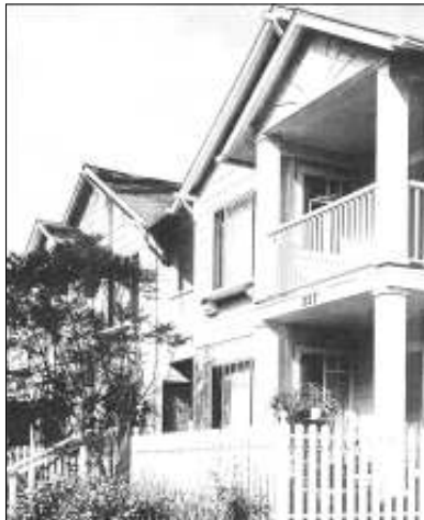
Cottage Gardens is a 17-unit affordable senior apartment complex built with federal low income tax-credit financing.
